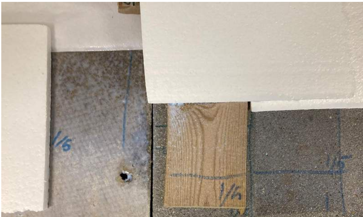
Photo 3 the sheets are sprayed with asbestos sealant.
