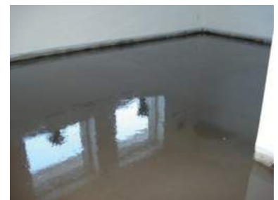
The finished Radon protection after only 24 hours
