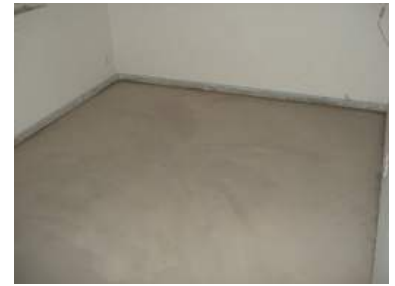
Floor before Radon protection
