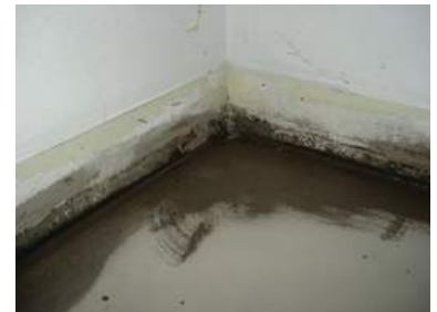
Edges and floor are sealed
