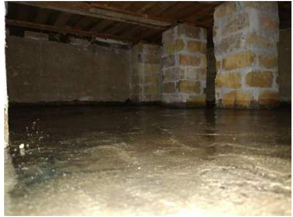
#4 Terrain tires i crawl space able to be treated accordingly.
